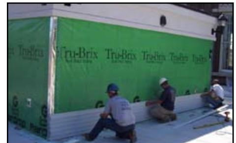
Installing the steel rails
