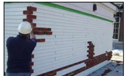
Installing the Tru-Brix tiles
