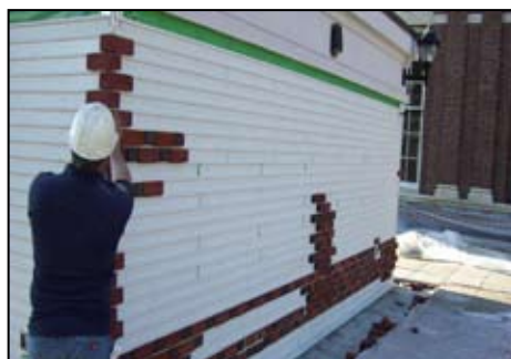
Installing the Tru-Brix tiles
