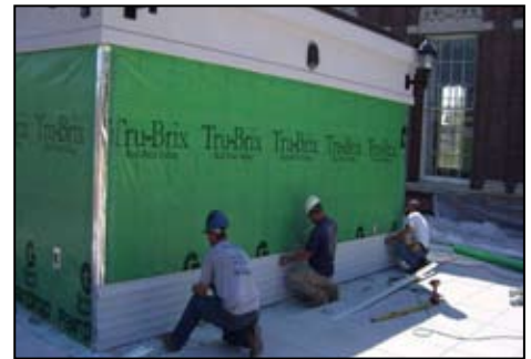
Installing the steel rails
